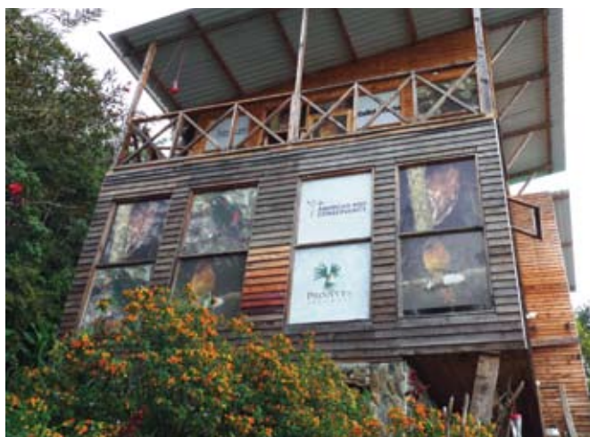
CollidEscape film applied to windows of the visitor's lodge at El Dorado Reserve in Colombia, January 2009. This see-through film keeps birds from colliding with windows. Photo: Fundacion ProAves, www.proaves.org
