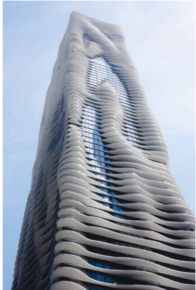
Chicago's Aqua Tower, designed by Studio Gang Architects, minimizes the use of reflective glass, making the 859-foot tower an excellent example of design that is both bird-safe and attractive. Photo: Tim Bloomquist
